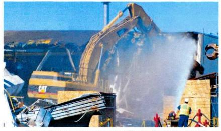
Heavy cutting equipment was used on the 333 Building to minimize worker risk and accelerate the demolition schedule.
